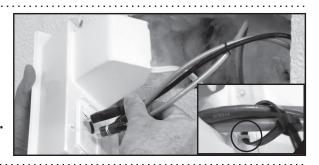
C) Slide PowerOUT panel into wall opening.
